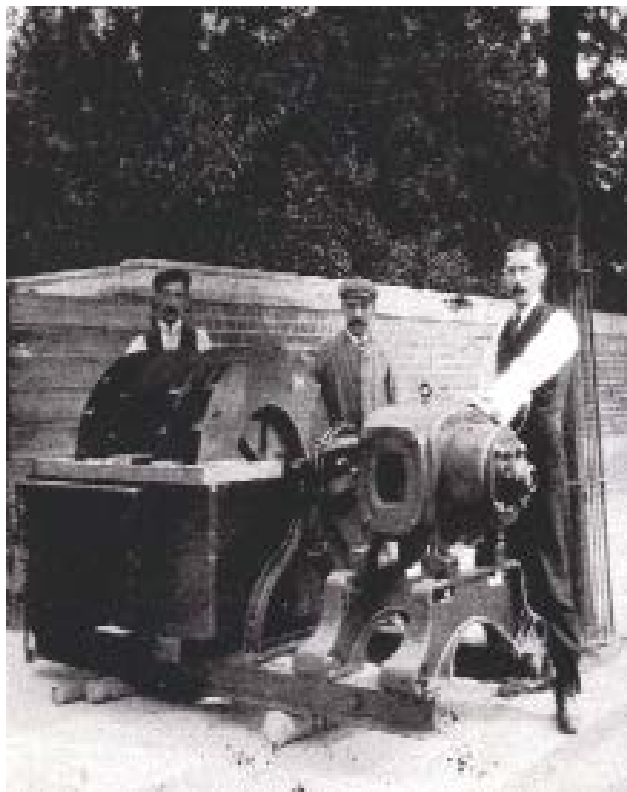
The arrival of the Kinetic blower in 1904 – after more than a century of constant service, it is still in use today
